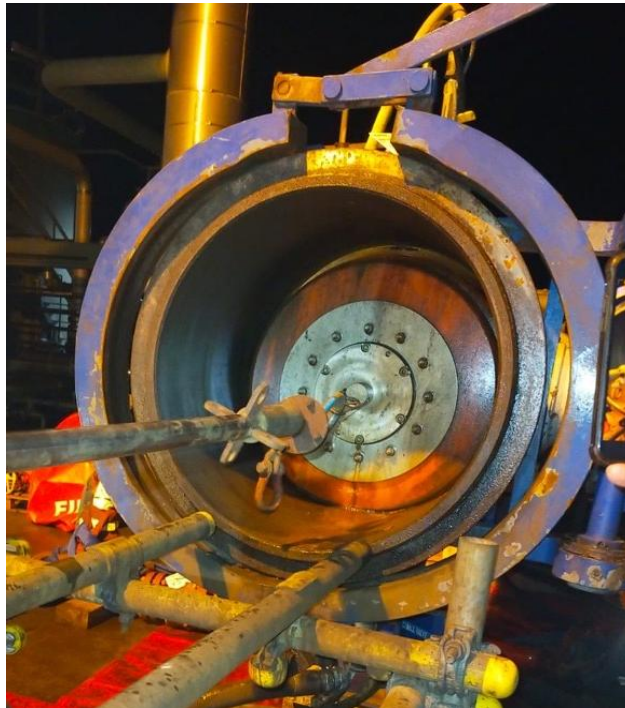
Figure 8: Final pig run. As can be seen, minimal residue and debris is evident.
