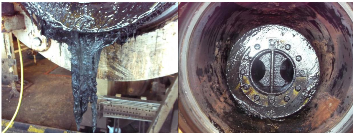
Figure 2: A very heavy and viscous residue was recovered by the initial Bi-Di pig runs.
