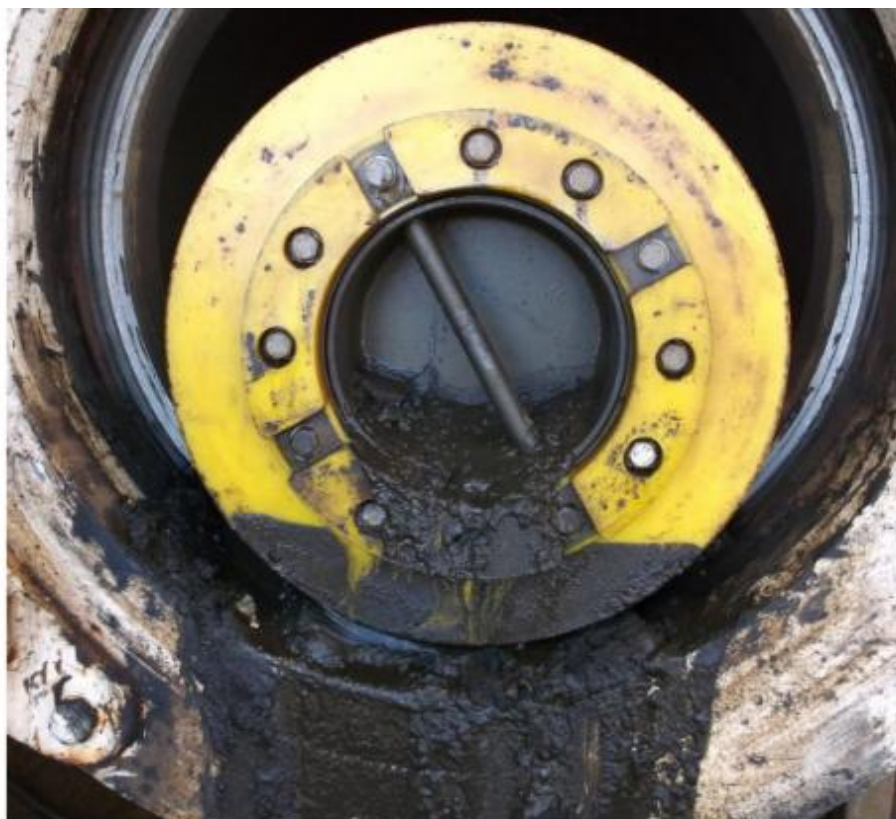
Figure 4: The demineralised water trains continued to remove significant residue and debris from the pipeline.
